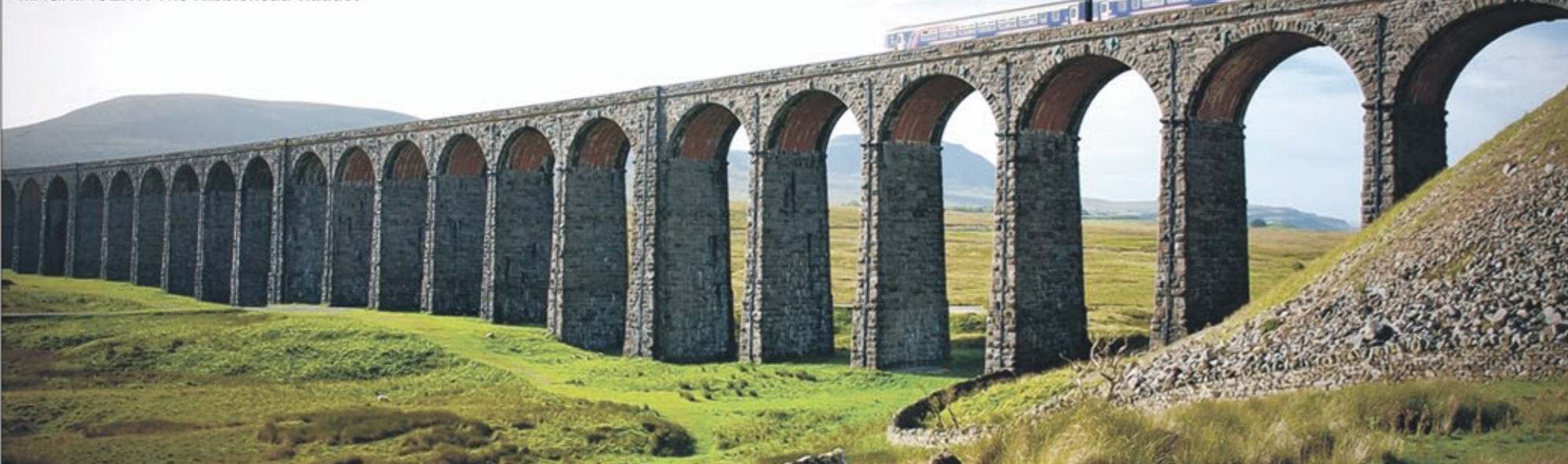
MAGNIFICENT: The Ribbleshead viaduct
